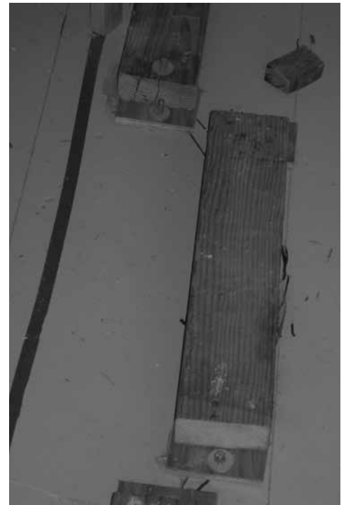
Anchor points were secured to the floor with powder-actuated anchors (.22 caliber). Additional blocks were added to raise the nominal 96" plywood sheets to reach Bruce's 99"-high ceiling. Dark strip at left is tape used to roughly define benchwork edges, partially-obscured wavy line set the desired curves of the Thin Wall.
