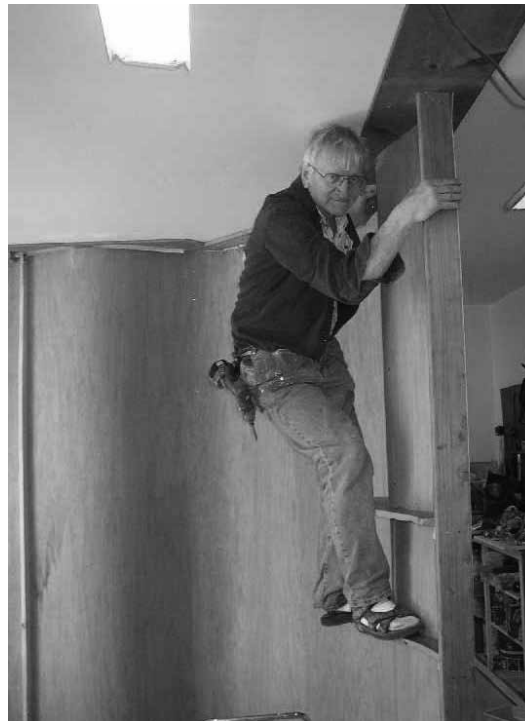
Walter Naumann shows that he's confident of the strength of Thin Wall construction by climbing on the first installed section. His feet are on the stiffening ribs set just below the layout's planned levels. Note also the wide boards screwed to the ceiling to provide convenient places to mount the upper anchor ribs. Two photos by Bruce Morden.
